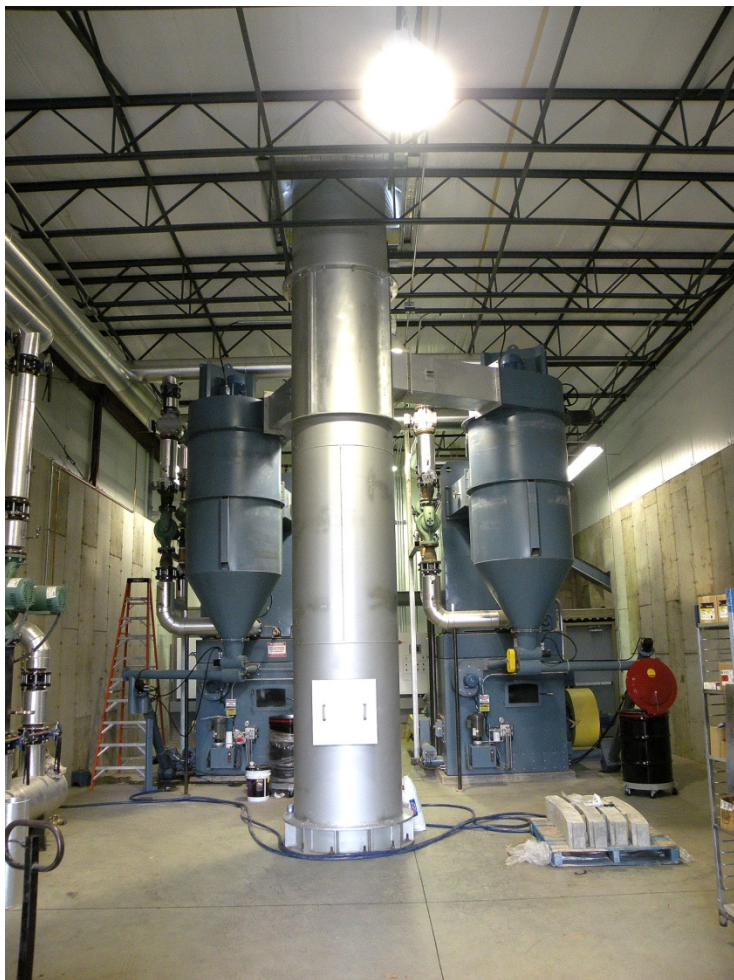
Geremia Greenhouses, Wallingford, CT --- Two 5,800,000 btu/hr 30# Hot Water Units
