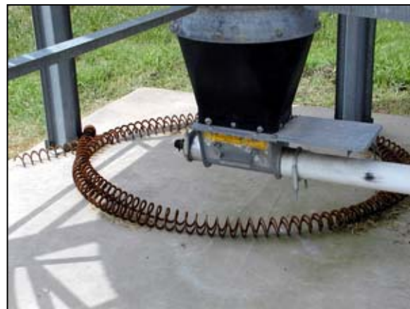
Figure 37: silo hopper bottom with tube auger (and extra open coils)
