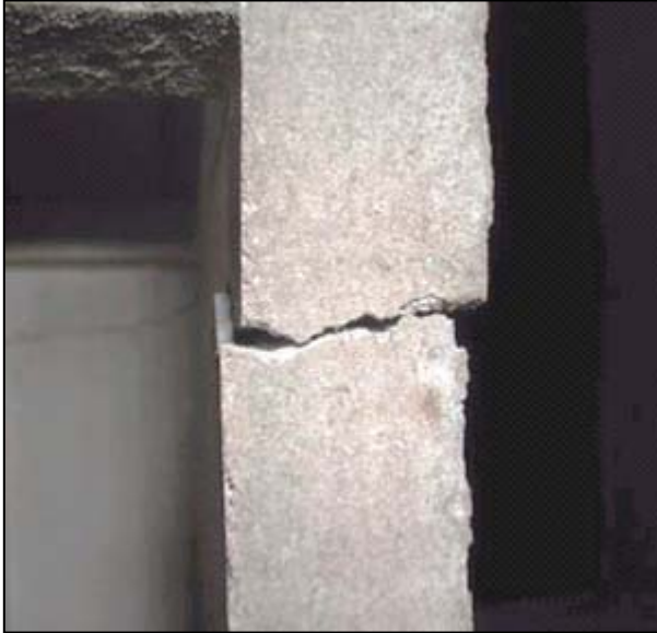
Figure A.3.7: Cracks in ceramic components
