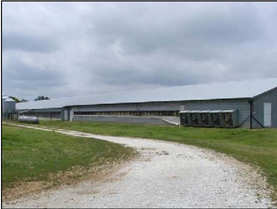
Figure 15: Broiler house reflecting older style tunnel ventilation design (curtains are closed during operation)
