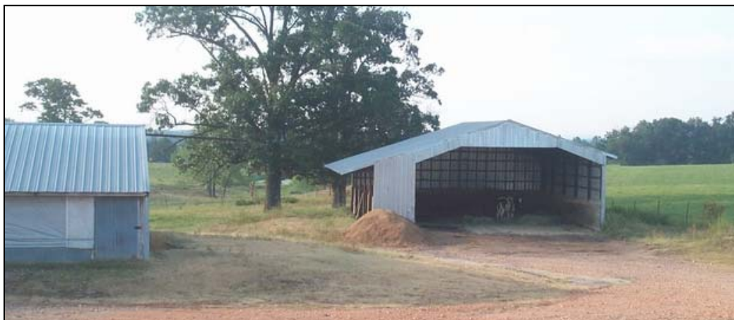
Figure 39: Litter Stacking Shed The building on the left is a broiler house.
