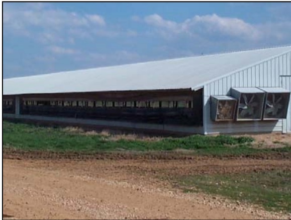
Figure 11: Broiler house using open sidewall drop-curtain design
