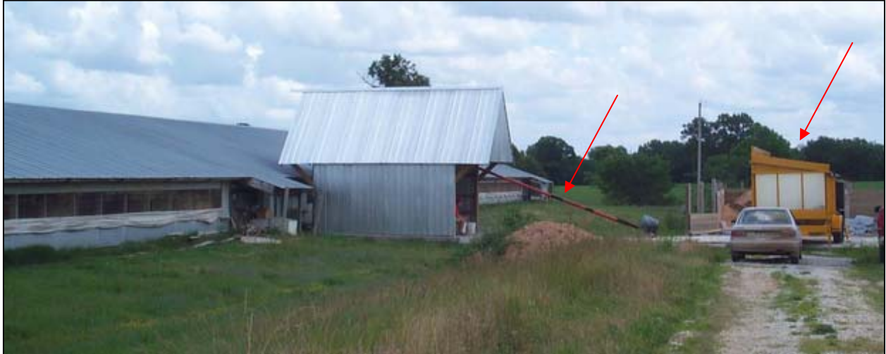
Figure A.2.2: Fuel bunker
